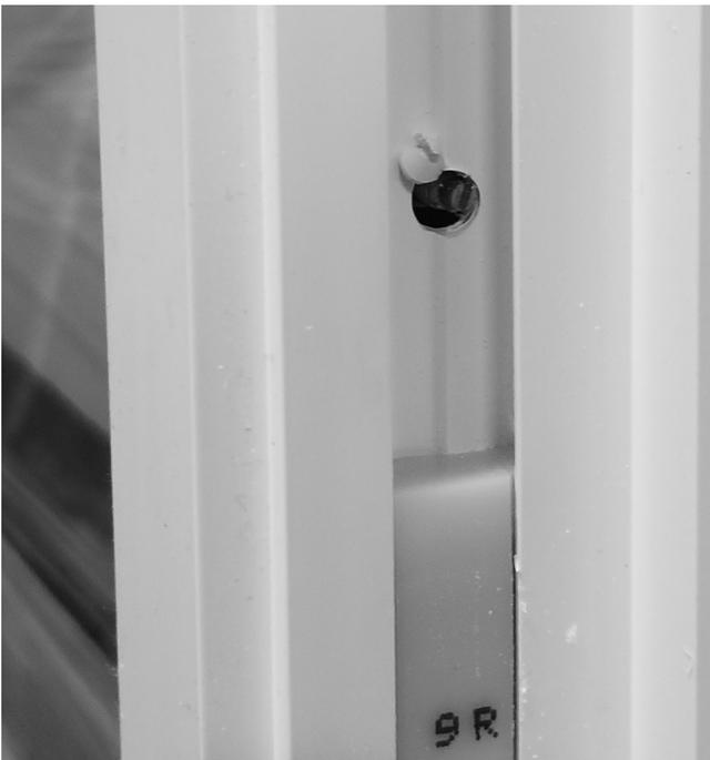
**STEP THREE:** Once all installation screws are driven, tighten wafer head jamb adjuster to bring jamb parallel with glass inserts. Repeat procedure on other jamb. Adjust as necessary.
