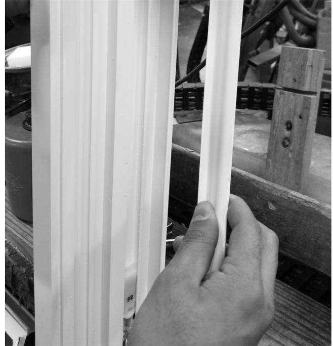
**STEP TWO:** Once unlocked, remove covers from jambs. Installation screw holes and wafer head jamb adjuster screws are now exposed.
