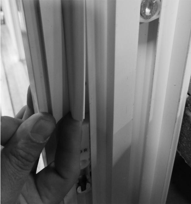
**STEP ONE:** To access wafer head jamb adjuster, lift lower exterior edge of balance cover side corners. Once started, it can be unlocked by sliding finger up jamb between cover and jamb.
